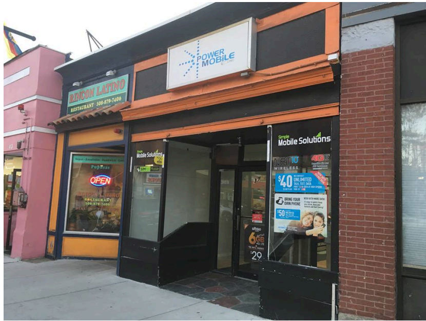
Power Mobile Before
