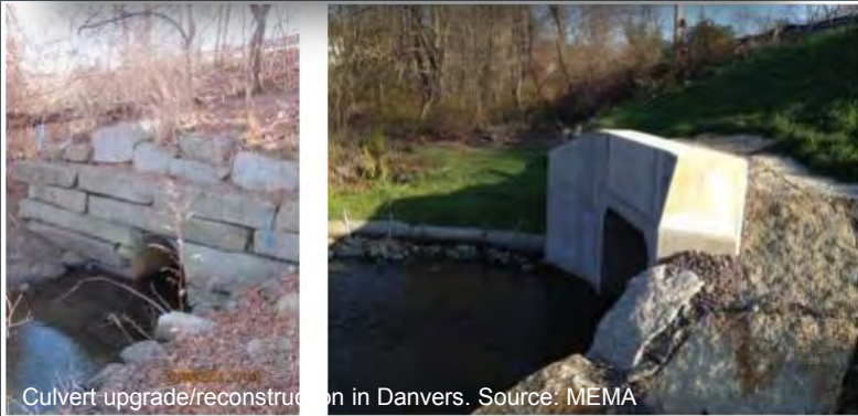
Culvert upgrade/reconstruction in Danvers. Source: MEMA
